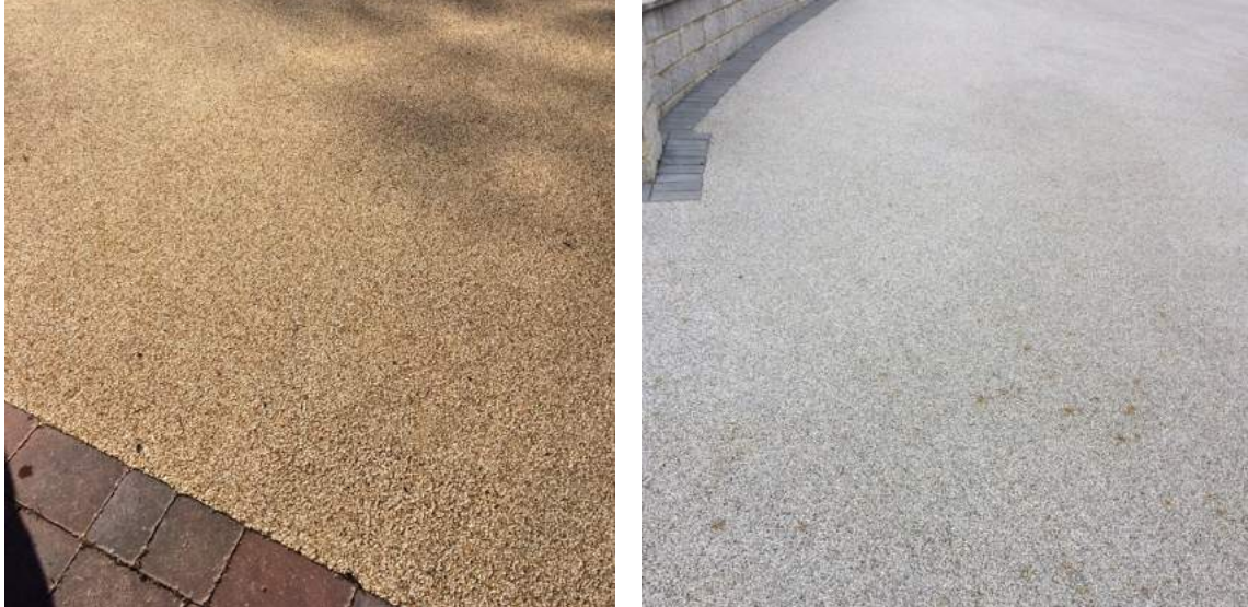
Figure 11: Examples of impermeable hardstanding (source: Google Images)
