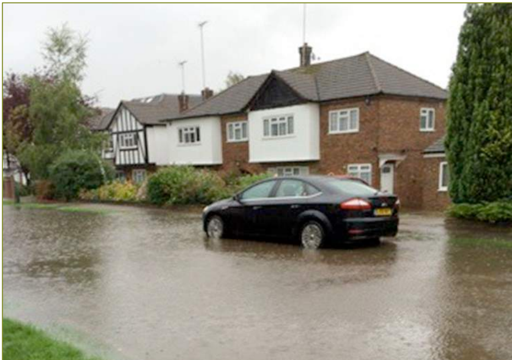
Figure 26: Flooding in Parkgate Crescent, 2015 (source: HWNPF)
