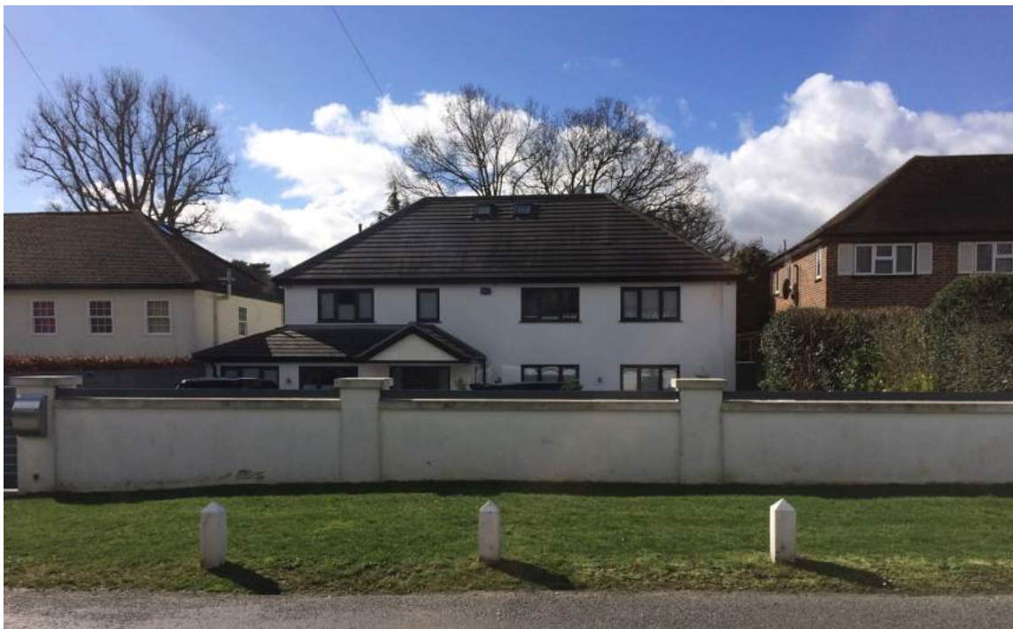
Figure 8: Example of boundary wall that adversely impacts on the quality and character of an area (source: Google Maps)
