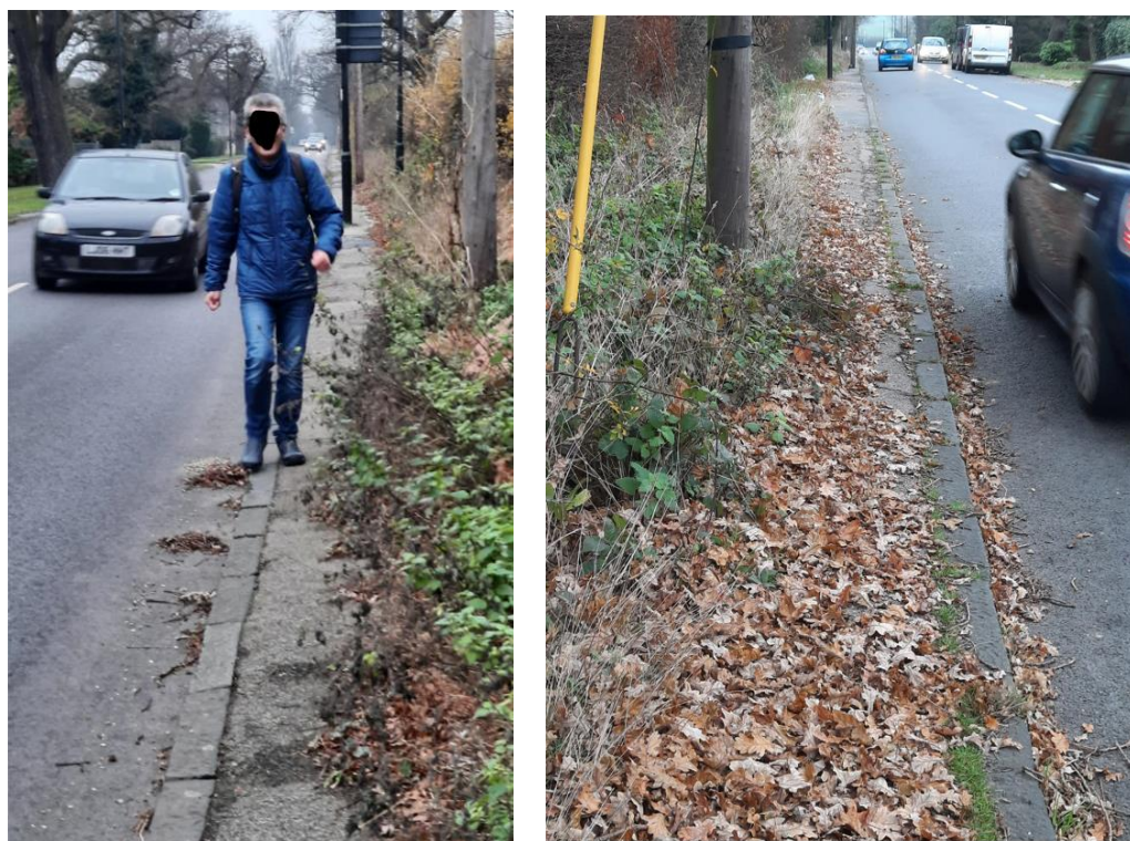
Figure 59: narrow and obstructed footpath along Waggon Road (no pavement on other side of road)
