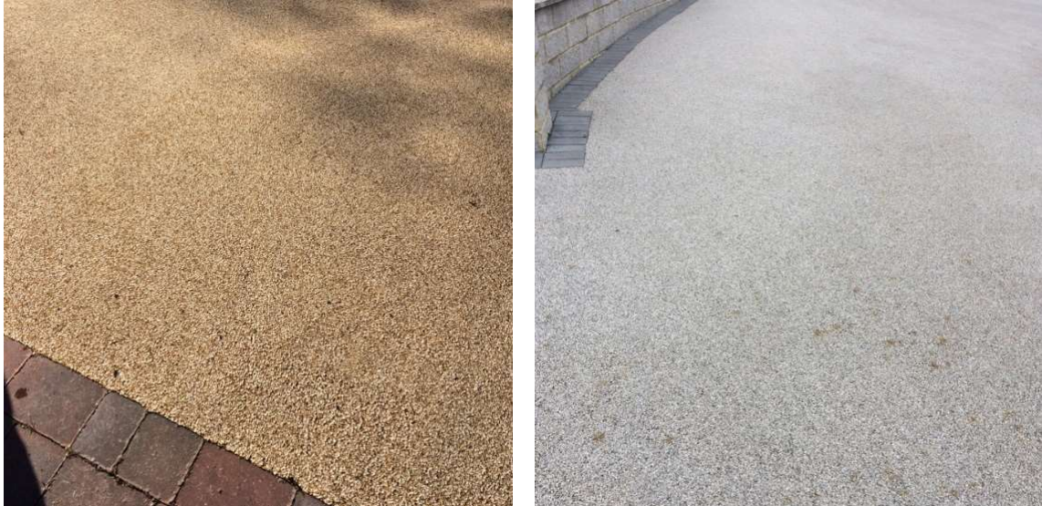
Figure 11: Examples of impermeable hardstanding (source: Google Images)
